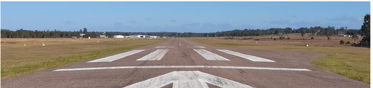
Runway 23 threshold, July 2023.
