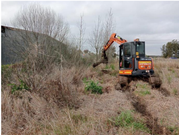
Removed a length of rotting fence which was leaning heavily into the open drain, to allow for easier removal of vegetation from the drain & behind the buildings.
