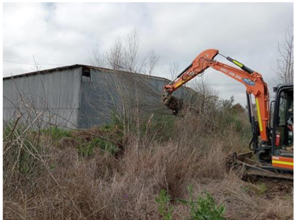
Removed a length of rotting fence which was leaning heavily into the open drain, to allow for easier removal of vegetation from the drain & behind the buildings.
