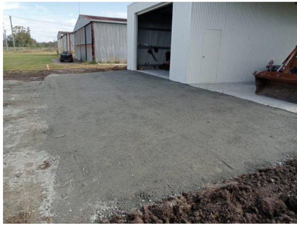
Cement stabilised road base ramp to full width of the Equipment Shed.
